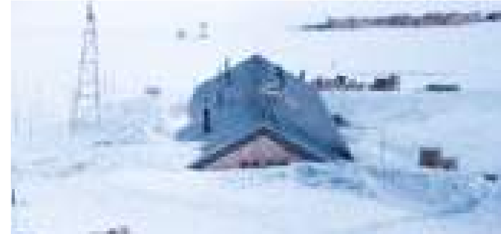
3 — Halley II Station's Access Points were entirely buried, forcing abandonment
