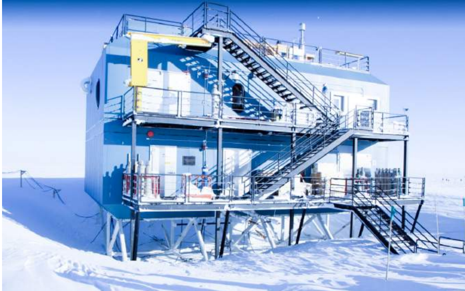
3 — Atmospheric Research Facility (ARO) — Meteorology Observatory
