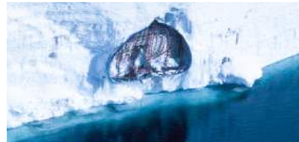
4 — Unable to rise above the rising snow, Halley III was buried, and has fractured into the Ocean
